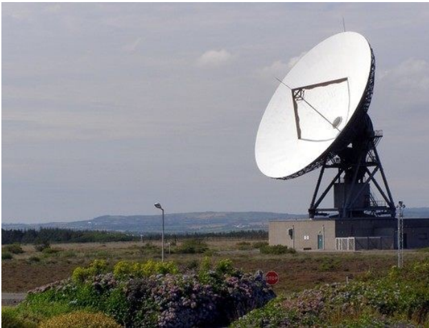
68. Goonhilly Earth Station
